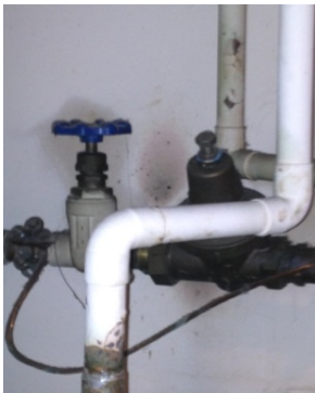
Photo 1 Water Shut Off Valve
