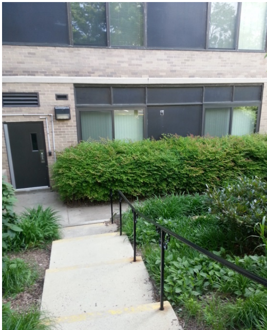
West Building concrete repair area
