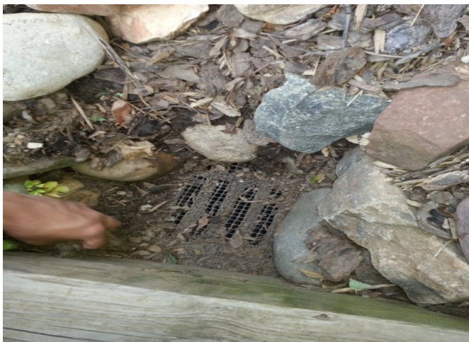
West Building clogged drain
